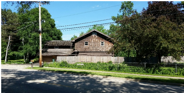
1018 Kilbourne Road June 2016
