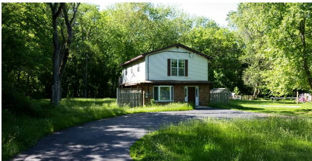
1001 Kilbourne Road June 2016
