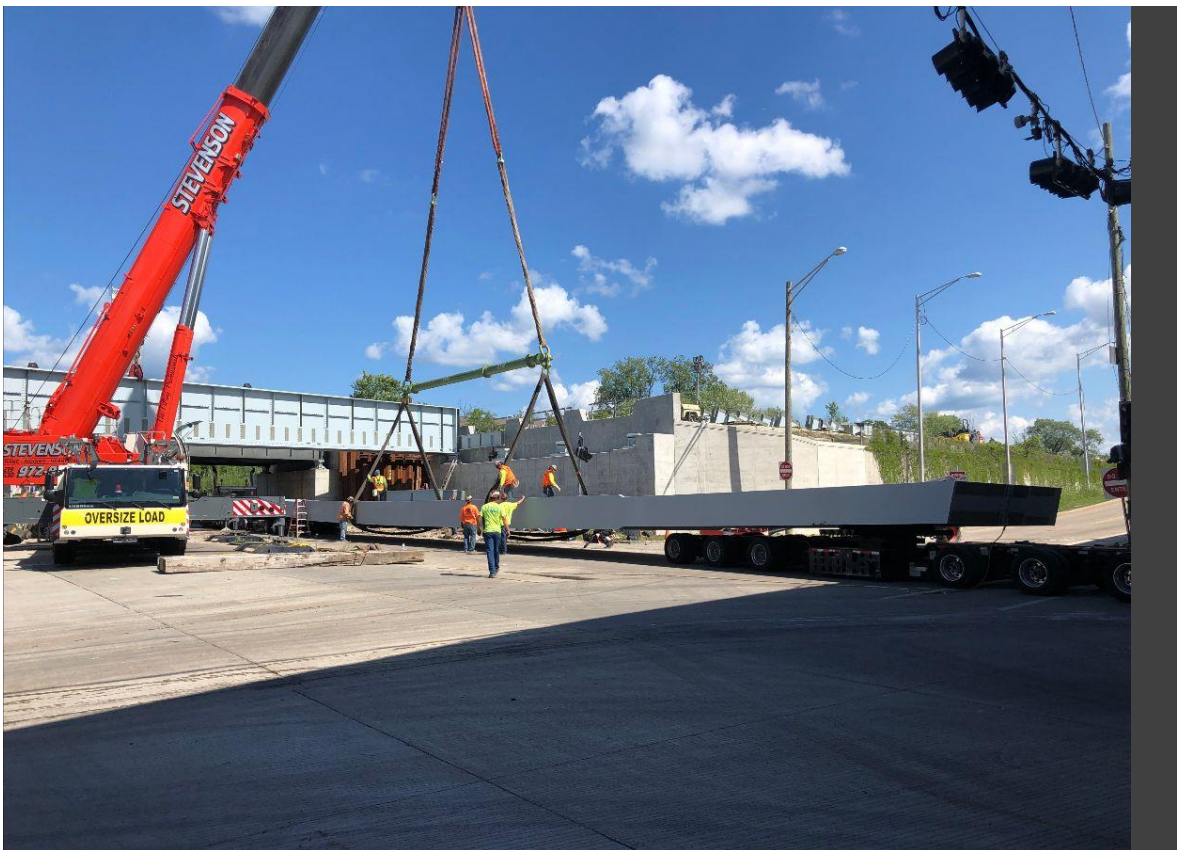
Beam installation at US-41 and Grand Avenue
