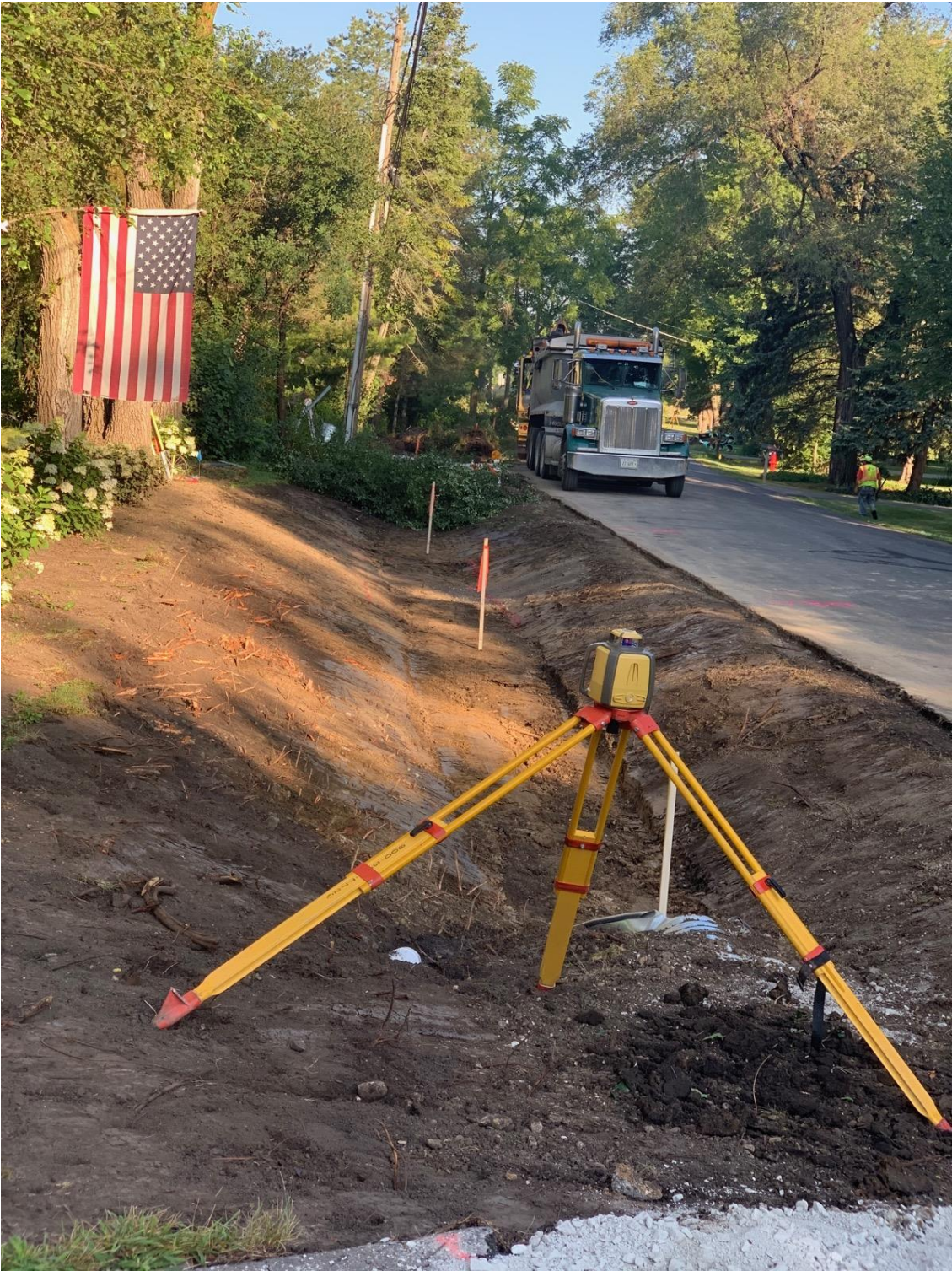
Drainage improvements along Elm Road
