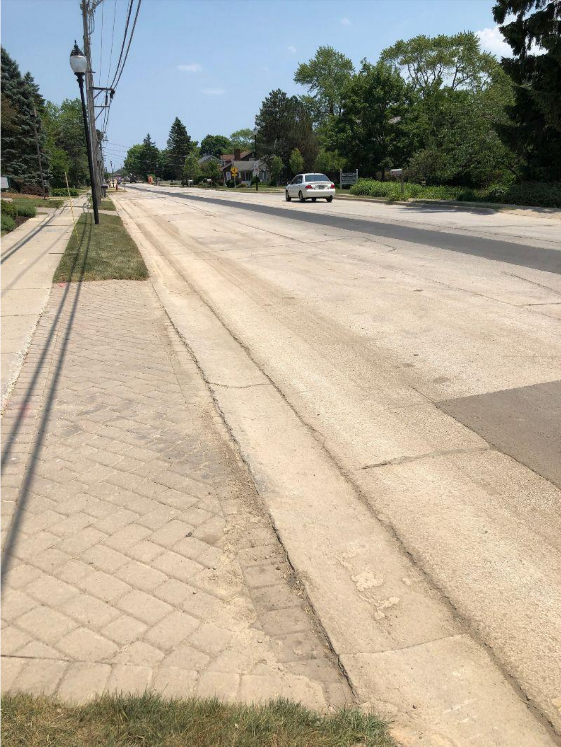
Main work on a section of Old Grand Avenue
