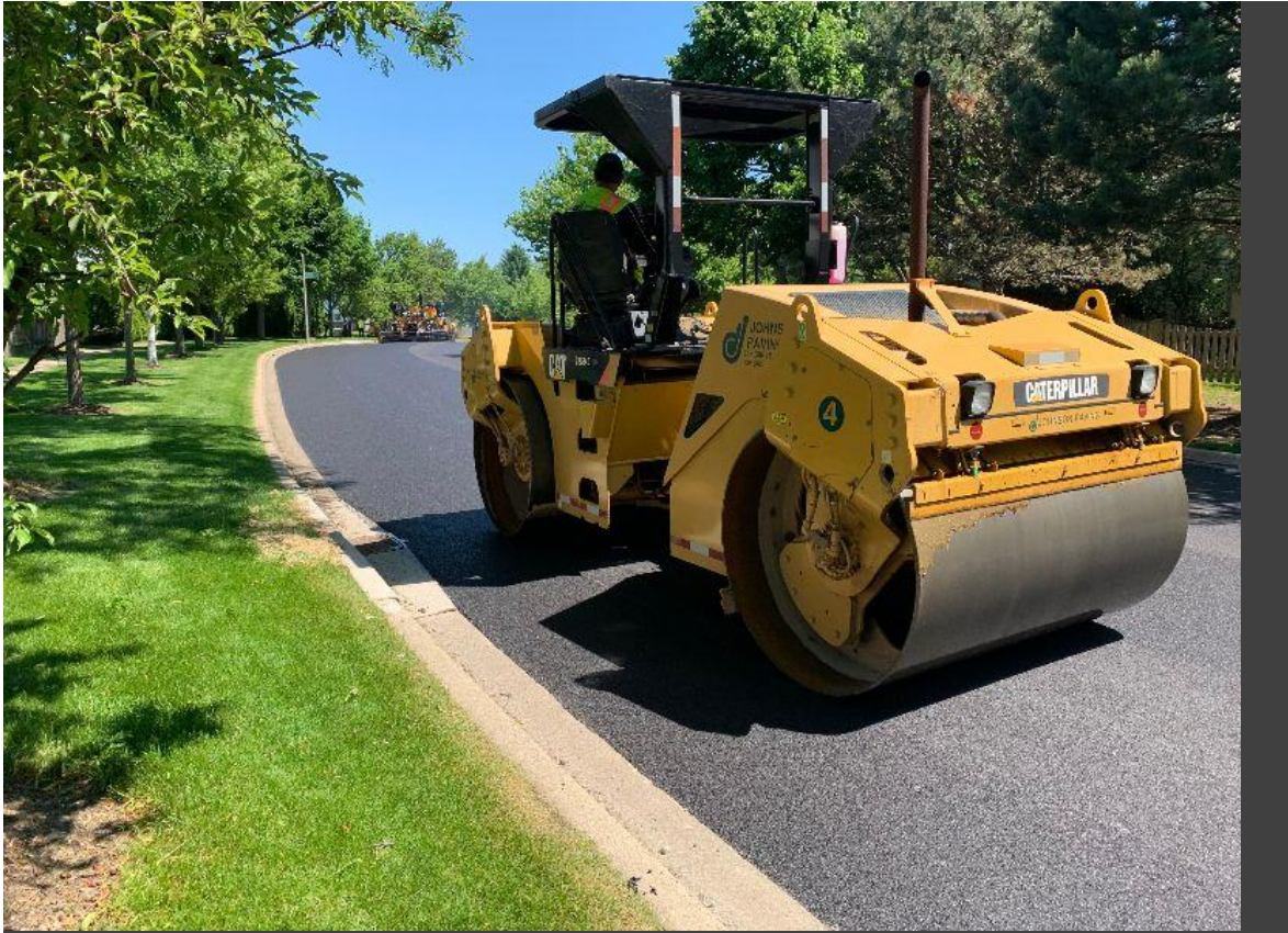
Crews completing paving of a roadway.
