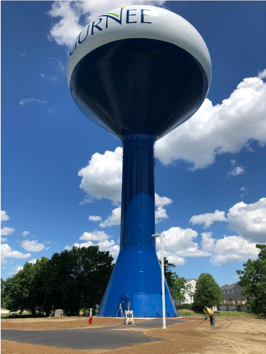
Knowles Road Water Tower painting is nearly completed. The final color will be blue, with a white band matching other Gurnee water towers. Knowles Road Water Tower #5 will be the first tower with Gurnee's new logo.
