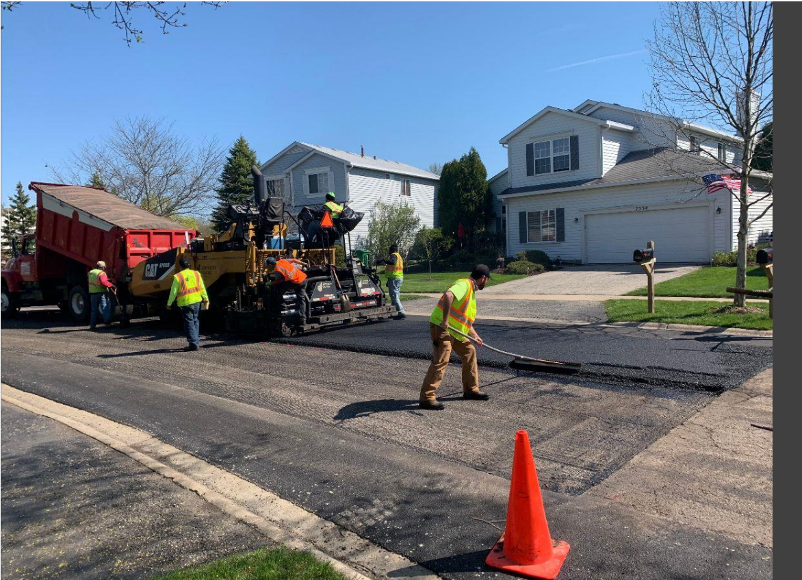
Crews resurfacing a section of roadway
