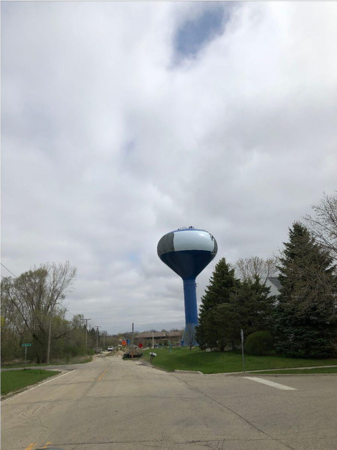
Knowles Road Water Tower is currently being painted. The final color will be blue, with a white band matching other Gurnee water towers. Knowles Road Water Tower #5 will be the first tower with Gurnee's new logo.
