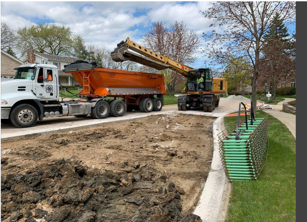
Crews removing a section of concrete roadway.
