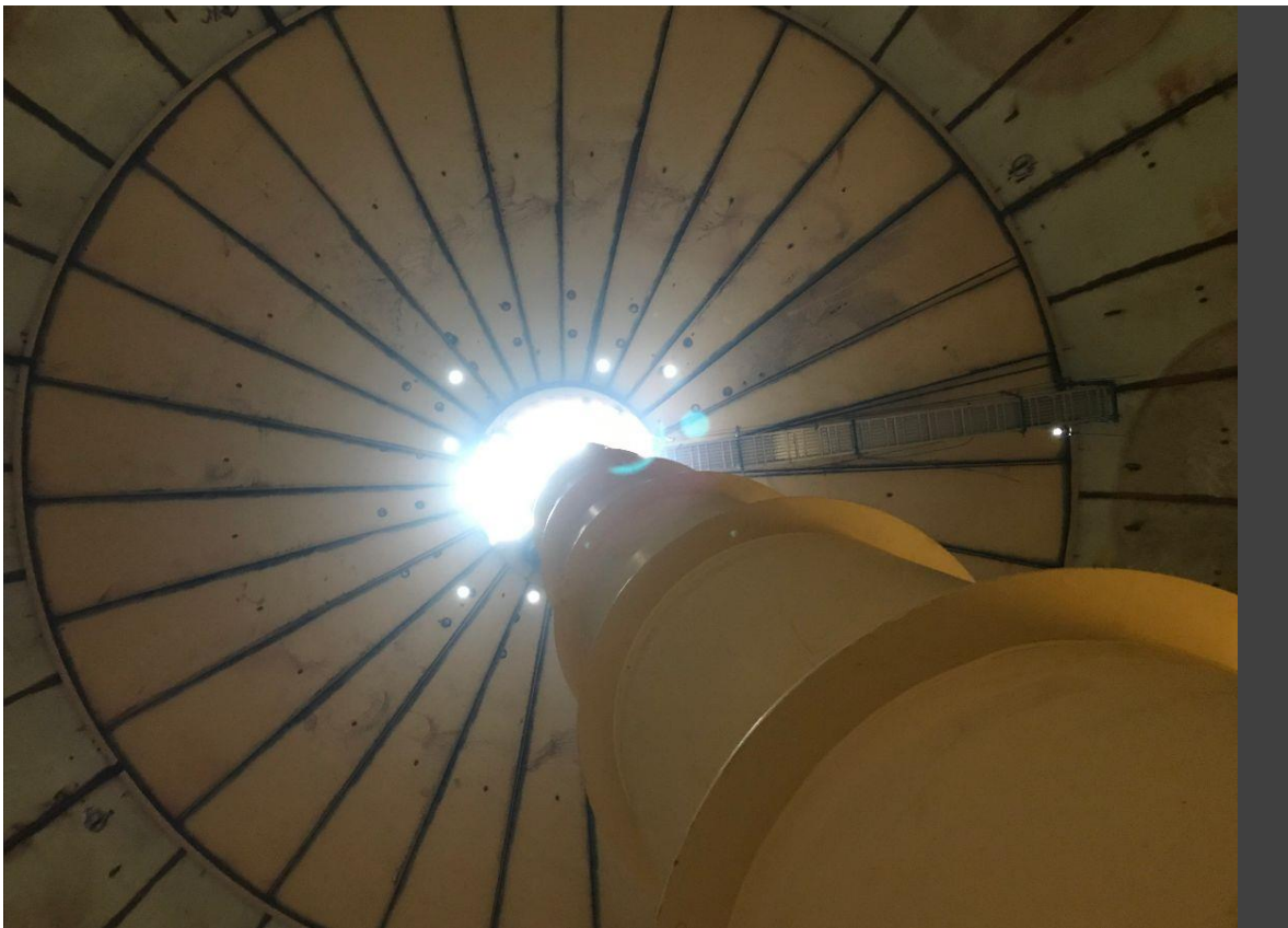
A view from inside the Knowles Road Water Tower
